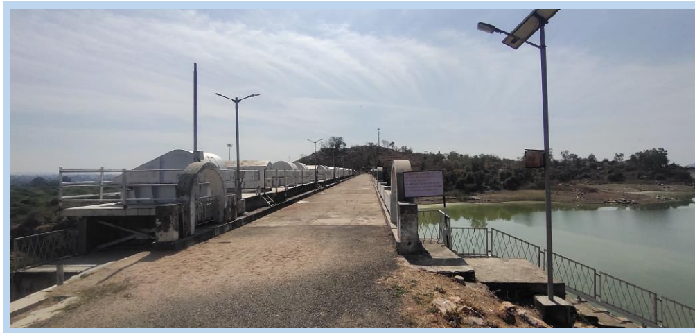
Dam Shutter Area
