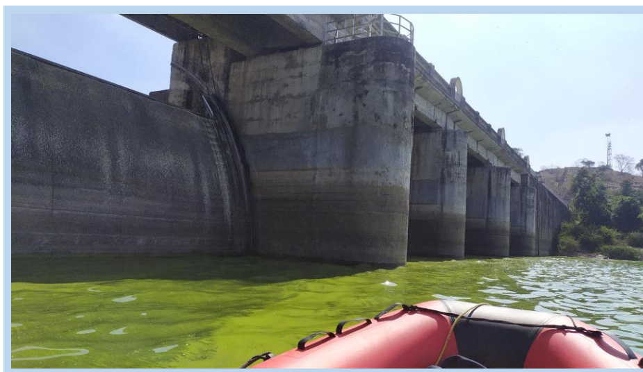
Survey carried out near Dam walls
